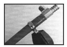
To remove the fittings, apply heat to the PEX tubing using a heat gun or hair dryer. Pull the fitting loose. Cut away the section of tubing that was previously clamped prior to continuing the installation.
