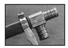
Place a flathead screwdriver under clamp tab and pry up to unlock.
